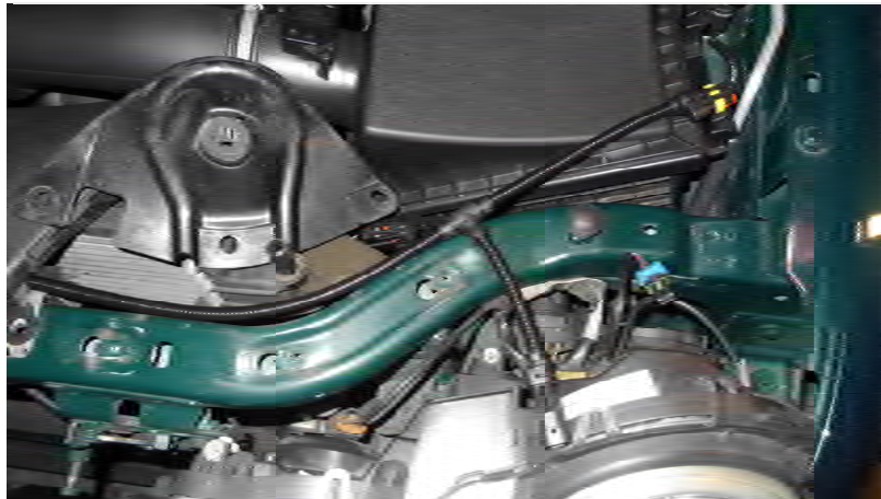
N/S main harness running below rad mount (shown removed). Turn signal spur will run below cross member.
