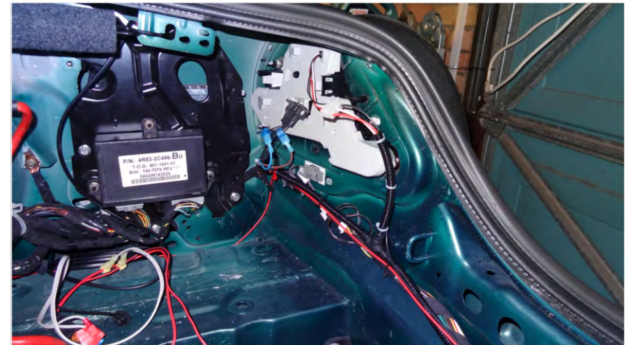
Connect Switchback LED to harness. Splice harness to lamp assembly connector (Off Side).
